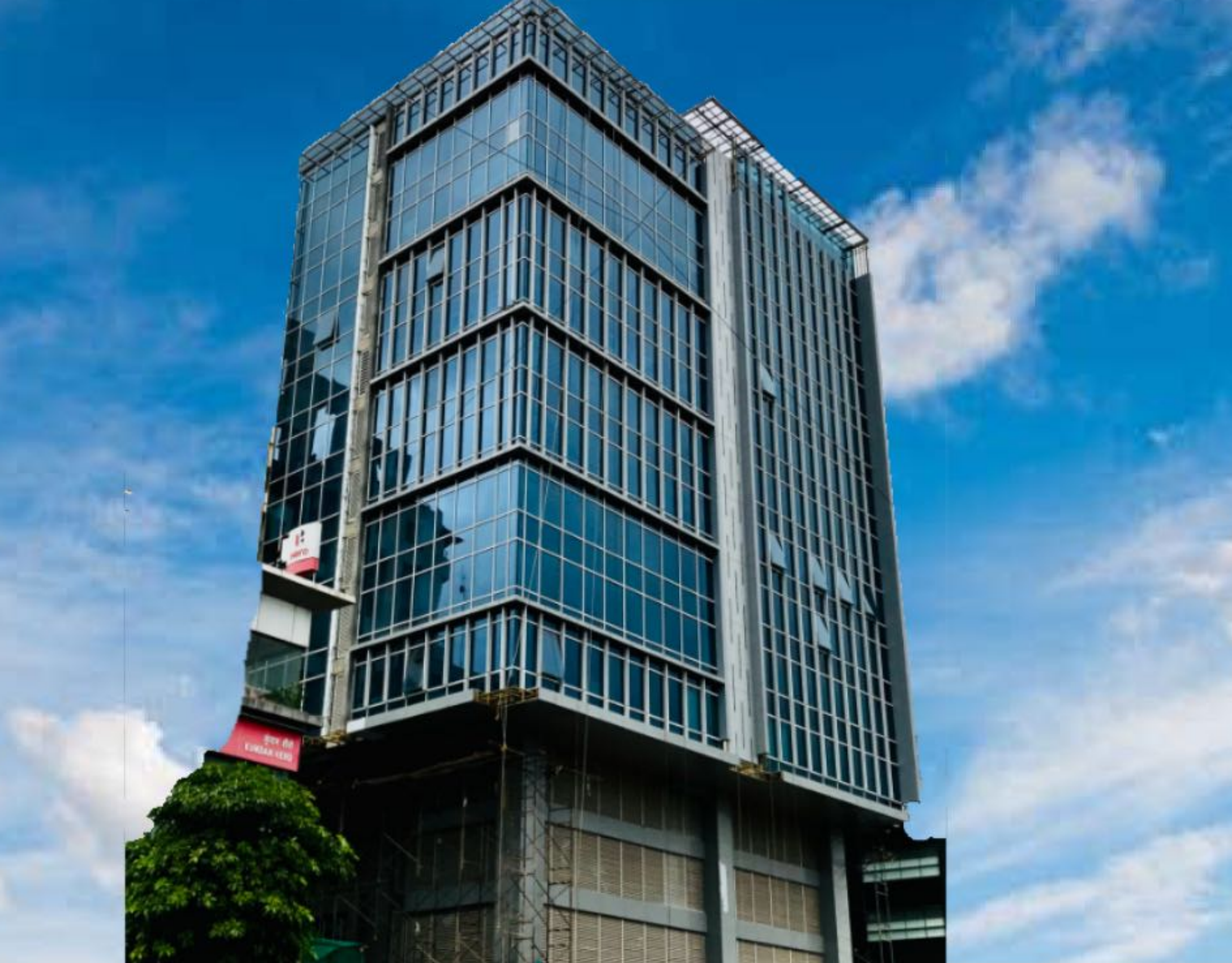
VANTAGE TOWER - Pune
